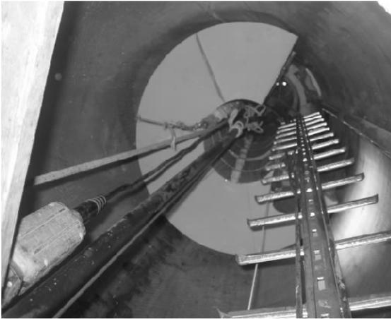
Figure 12: general view of the damper after site erection with permanent access using a safety ladder.
