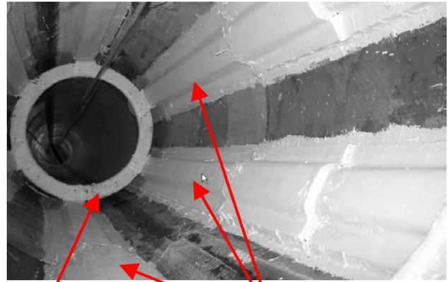
Circular stiffener at 30.950 m made of plywood protected by resin
