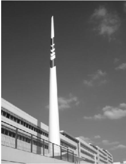
Figure 1 :The amplitude of vibration was observed to be as large as 1.200 m on either side of the mast.
